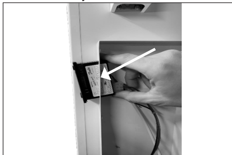
6: Push the thermostat out
