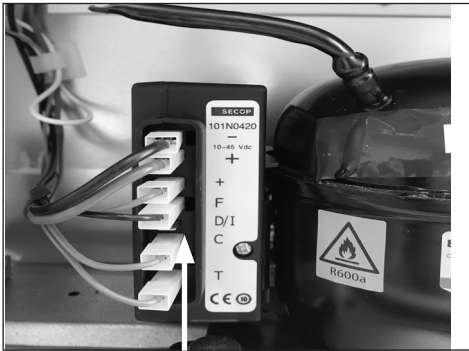
1. Dismount the 6 wires from ECU.
