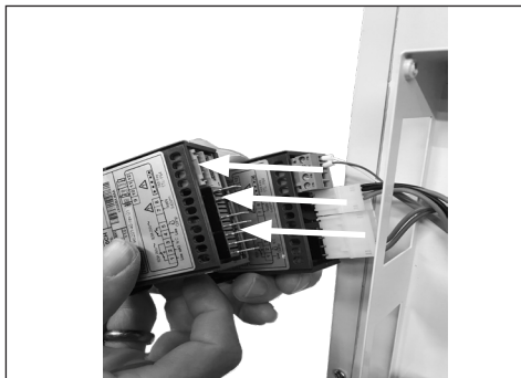
6. Switch the wires from old to new thermostat one by one
