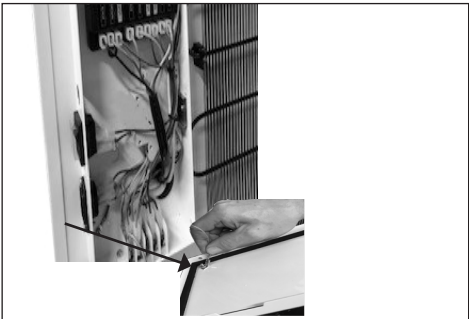
11. Remount grounding wire.
