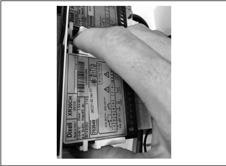
9. Use your finger to press/slide the back the fixing clamps to fasten the thermostat body
