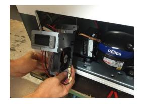
4: Push clip on left and right side and pull out thermostat
