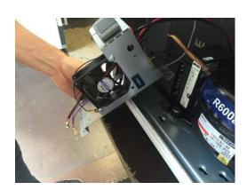
4: Loosen the 2 screws with a torx t20
