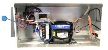
1: Loosen the phillips screw a couple of turns
