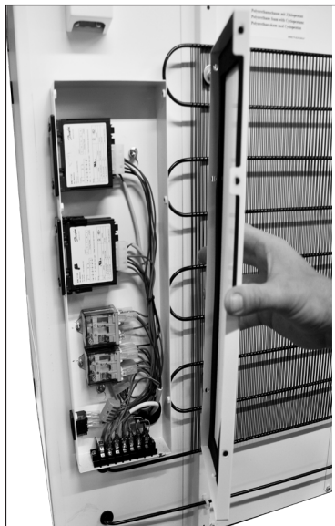
1. Access to electrical components Dismount 6 x Torx 20 screws and unmount the junction box lid
