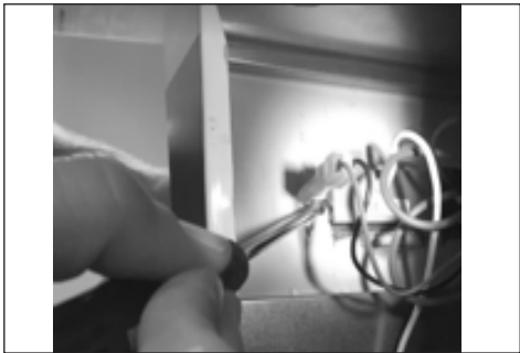
7. Use a screw driver to gently push the socket of the thermometer
