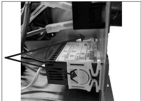
4. Remove the two clamps holding the thermostat in place
