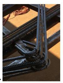
Place a reinforcement bar (N) in each corner of the braces (H). Raise the reinforcement braces one at a time and tie a string around each intersection – distribute the braces (H) evenly along the bars (N). When the frame is tied together, place the reinforcement U-braces (HH) on top of the assembly as shown below – the center square should be approx. 270x270mm to fit the anchor – see below. Finally tie a long string diagonally as shown below to make the basket rigid.
